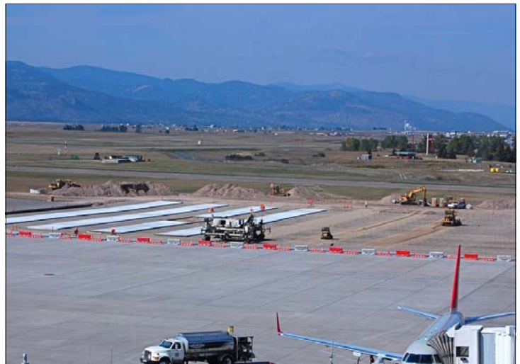
De-icing pad under construction, seen from the terminal.
