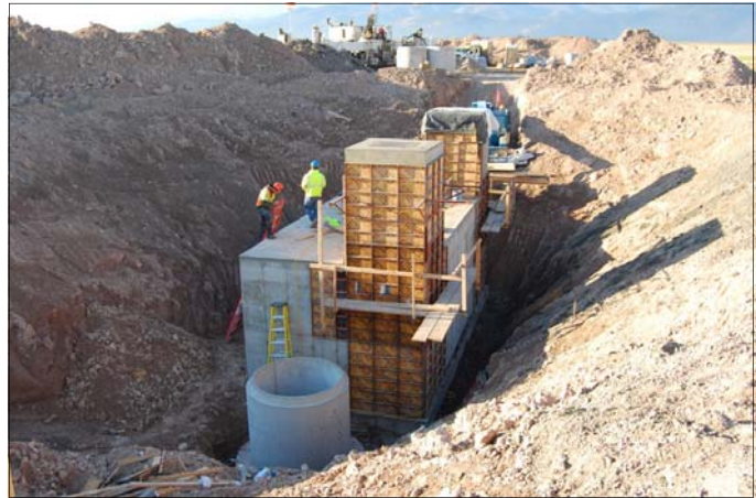
The house-sized storage tank, for used de-icing fluid, under construction.
