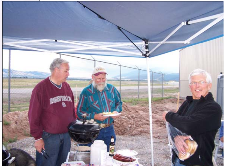
Left: Owners can enhance the interior of their hangars, as allowed by County building code. Hank Butzel measures not once or twice, but maybe lots more in his meticulous installation of ceiling and insulation.
