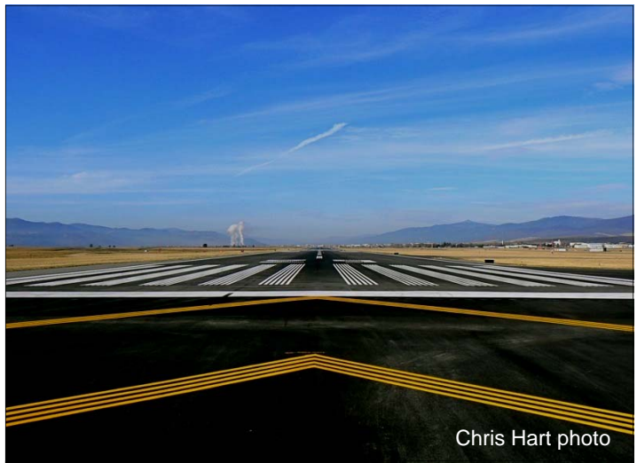
Full length view of the reconstructed Runway 29.
